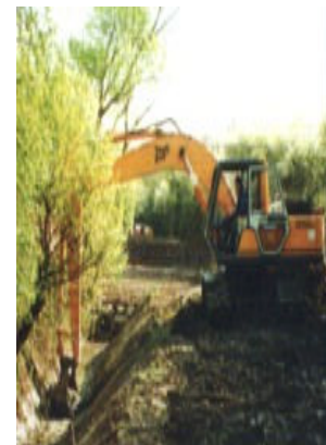
Land Drainage Works
